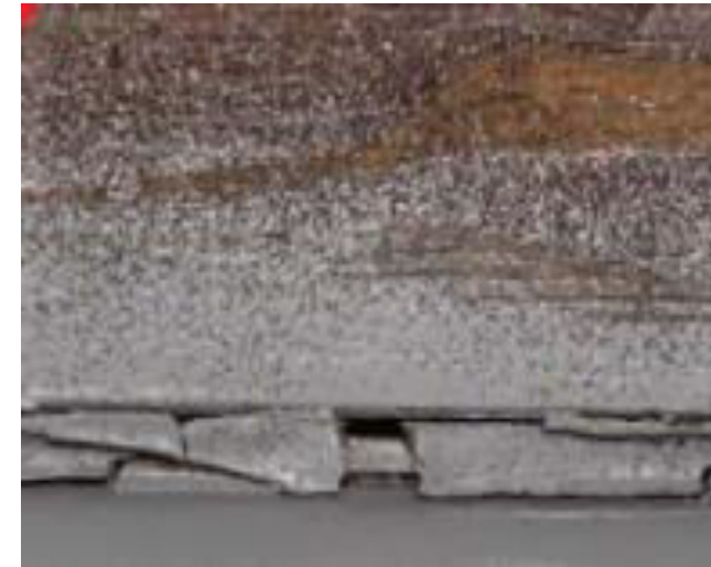
Sealant failure
